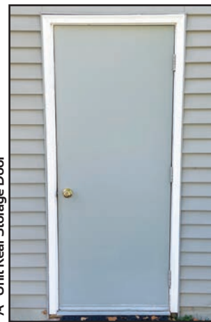
"A" Unit Rear Storage Door
