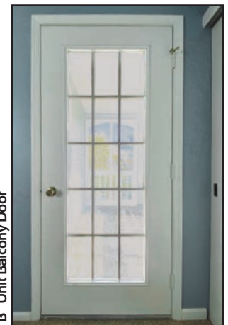
"B" Unit Balcony Door
