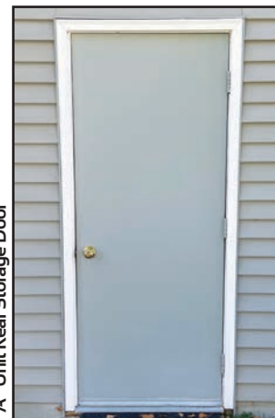
"A" Unit Rear Storage Door
